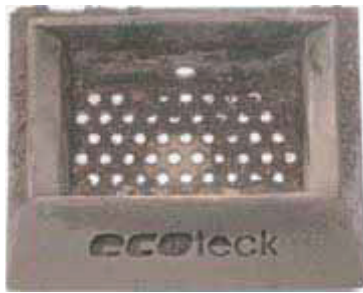
Burn pot liner needing cleaning with holes blocked by ashes
