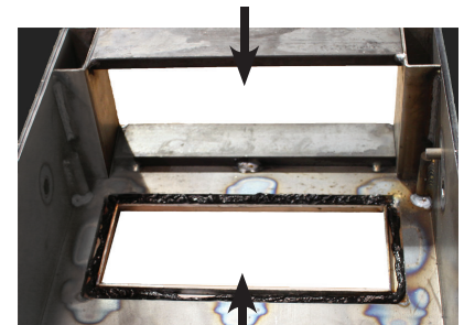
BYPASS DOOR OPENING
