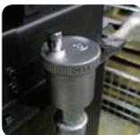
When filling the boiler, check that the Jolly valve (picture on the left) is working properly by venting the system. The maximum Loading pressure with COLD water should be of 1 bar.
